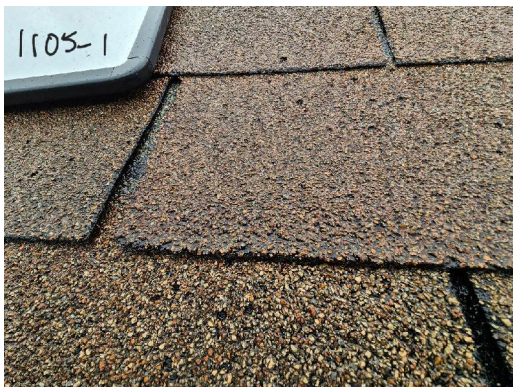
1105-1 Asphalt Shingle/Tar Typical Exterior Roof
