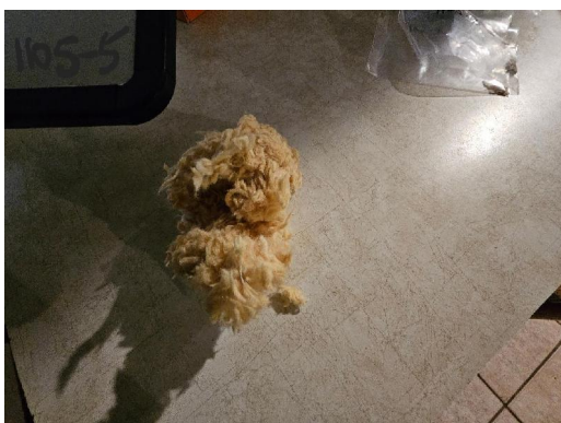
1105-5 Insulation Typical Interior
